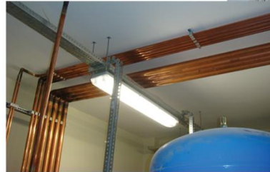
Esenguly Etraf Hospital, Turkmenistan, 100beds, turnkey MGS project, 2009
